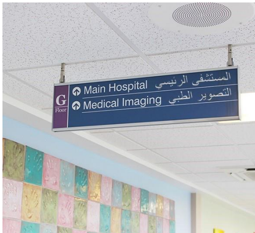
Figure 5.5: Corridor directional sign, ceiling mounted
